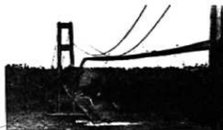
Figure 17.12: Collapse of Tacoma Narrows Bridge in 1940 during a windstorm.
